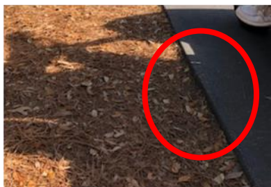
The above picture illustrates an area where a 1-2” drop off exists due to a lack of dirt and pine straw.
