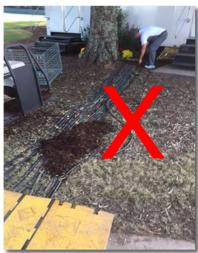
Properly secured and hidden cables minimize the risk of a trip and fall AND create an aesthetically pleasing environment for tournament guests.
